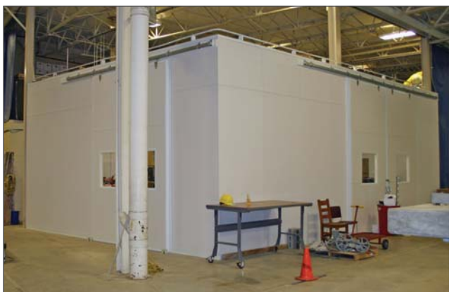
Figure 20. New room constructed in Highbay for ROV storage.
