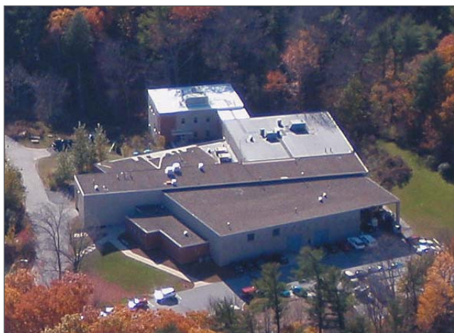
Figure 12. Aerial view of Chase Ocean Engineering Lab and the NOAA/UNH Joint Hydrographic Center.
